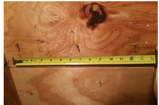
6 inch field nail spacing
