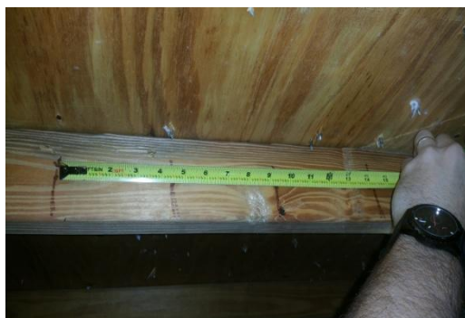
6 inch ridge nail spacing
